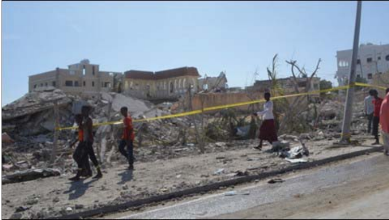
Figure 5: Damage to adjacent buildings.
